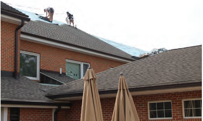
Roofers from Weaver Commercial used safety equipment as they installed new shingles on Village Townhouses.
